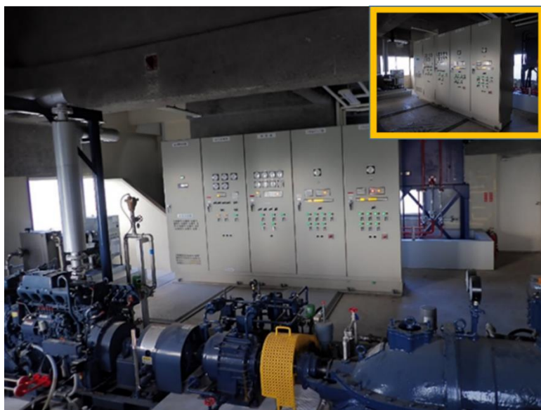
▲ Introduction of control system at a water treatment facility
