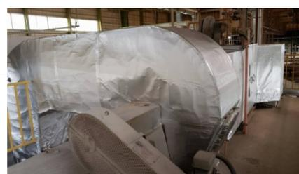
▲ We also have sheets to improve the thermal efficiency of machinery and equipment and to prevent dew condensation in refrigerator/freezer equipment.
