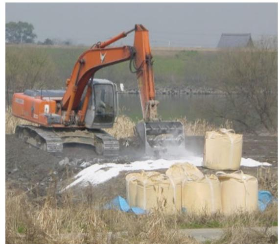
▲ The schwertmannite system insolubilizer with iron as the main material, and the hydrotalcite insolubilizer with aluminum and magnesium as the main materials. Anions are drawn inside, and cations are adsorbed on the surface.
