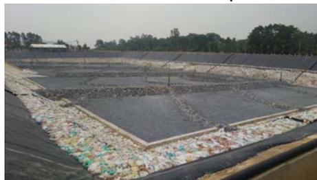
▲ Suppression of the generation of methane gas by aerobic bacteria due to ventilated structure of landfill
