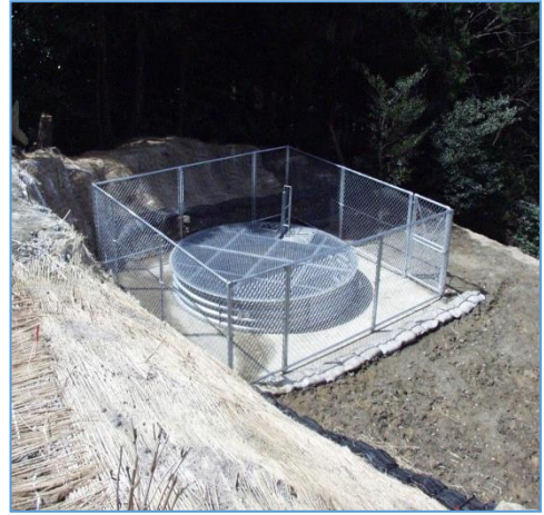
[地すべり防止工（集水井工）]
