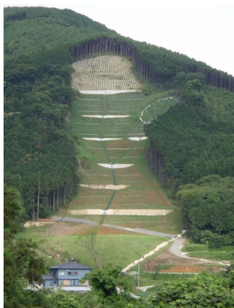
[土留工、法枠工]
